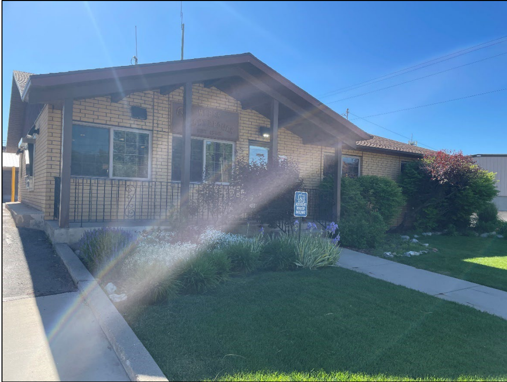
Front View of Main Building
