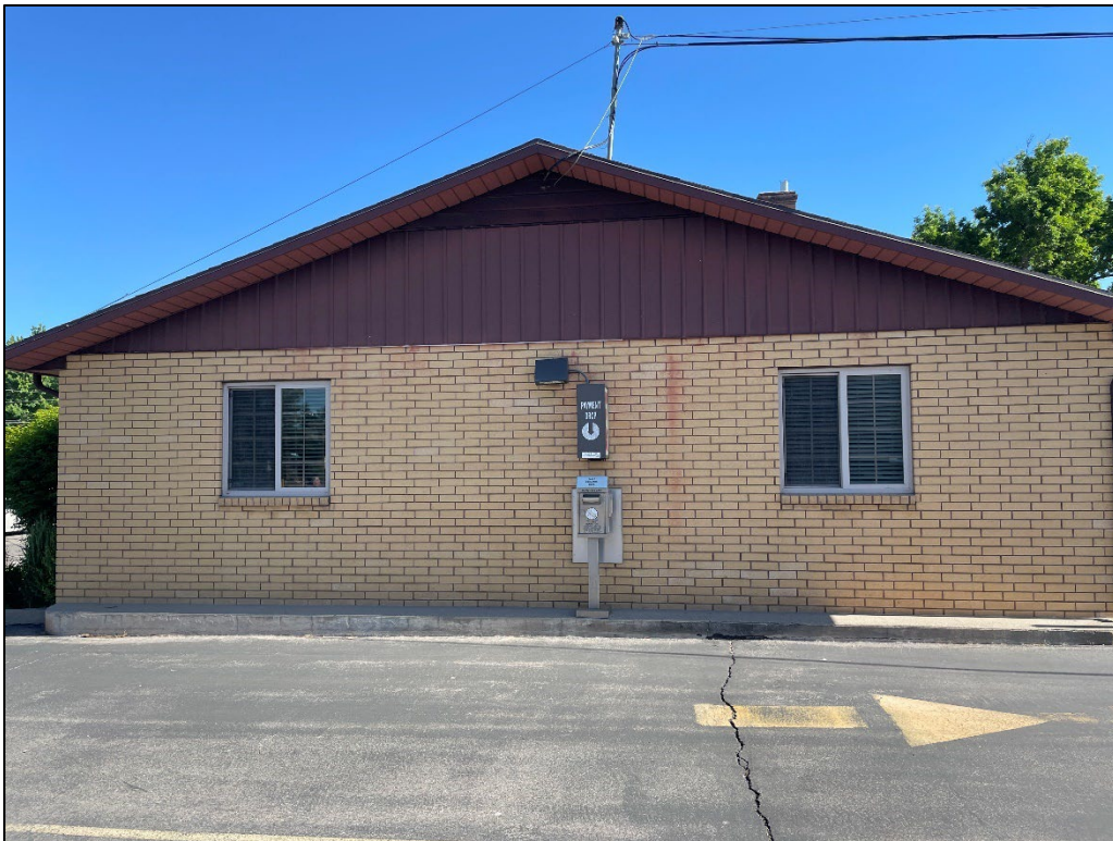
Main Building – South Elevation
