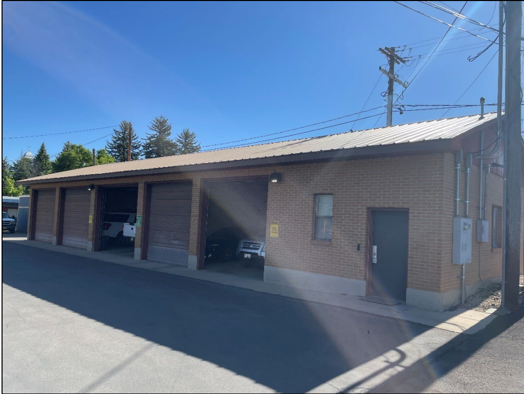
Front View of East Building
