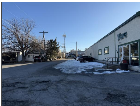
Northern façade of flex bldg.
