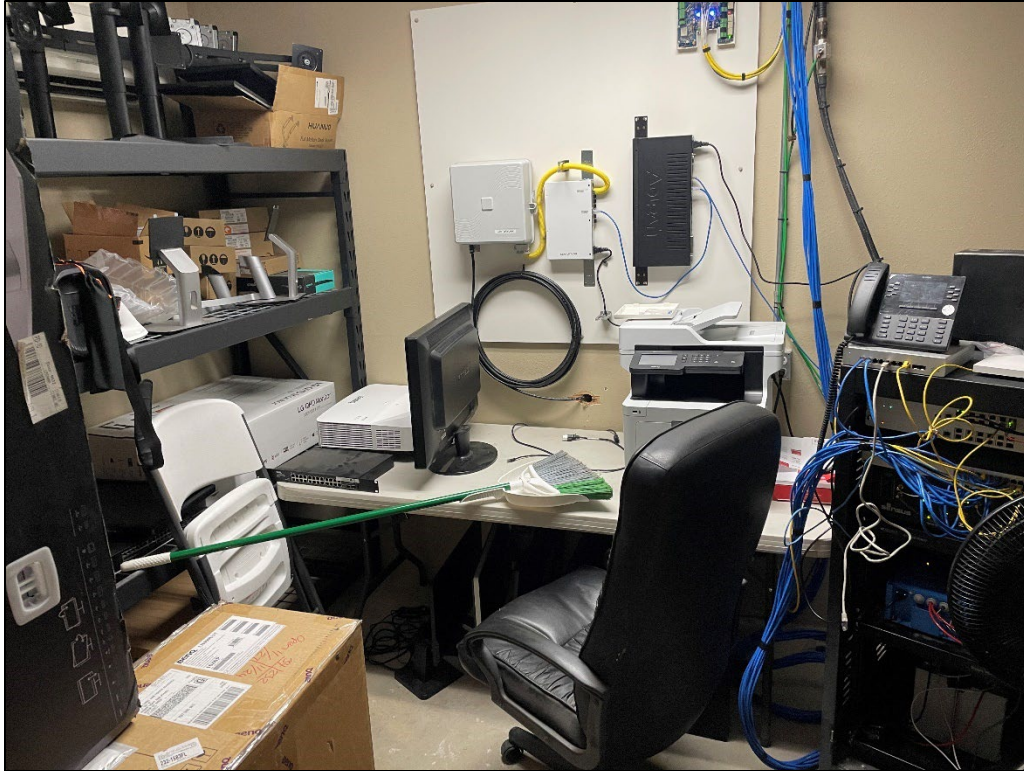
East Building Office Space
