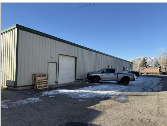
Northern façade of flex bldg.
