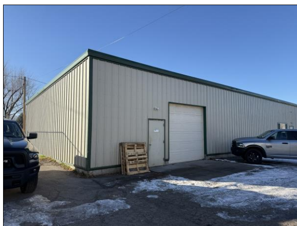
Eastern façade of flex bldg.
