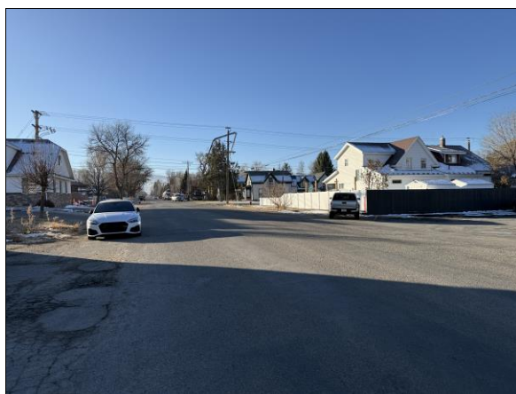
Looking south along 100 West (Sub. to left)
