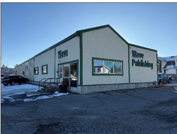
Western façade of flex bldg.
