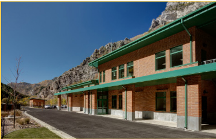
Ogden Water Treatment Plant building
