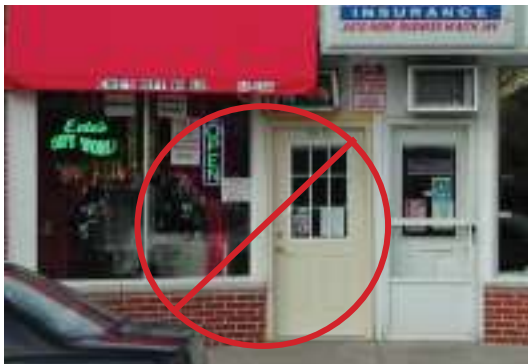
Prohibited: Residential Grade Doors on Commercial Buildings
