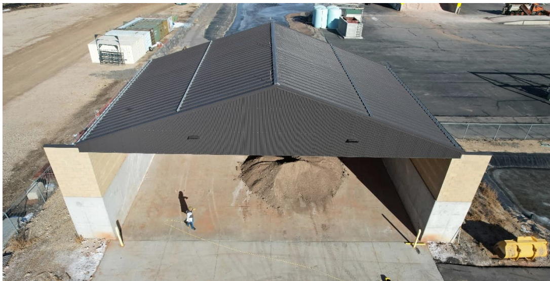
Figure 2. Front (south) elevation of subject structure.
