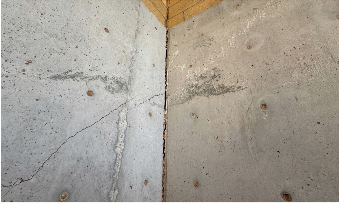
Figure 8. Interior northeast corner of subject structure.
