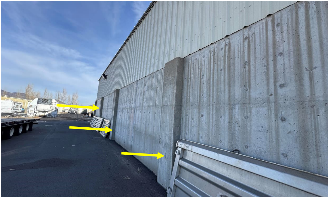
Figure 13. Piers constructed along exterior wall at UDOT salt storage structure.
