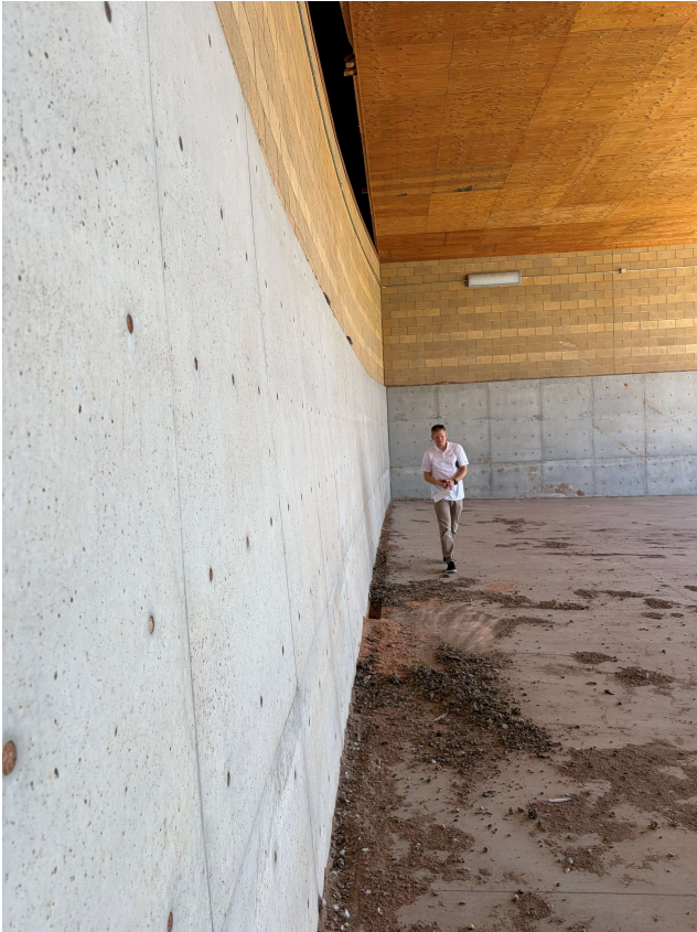
Figure 3: Back wall lifting & pulling away from floor Figure 4: Gap between ceiling finish and back wall
