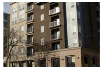
Figure 3.15 (5). Balconies Integral to Facade
