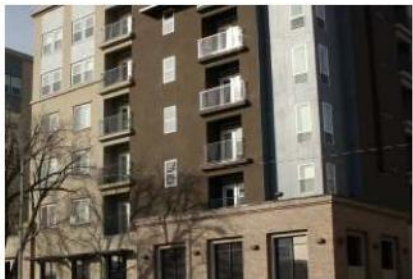
Figure 3.15 (5). Balconies Integral to Facade
