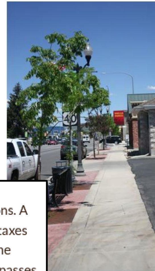
Fig 7: Existing Streetscape Conditions
