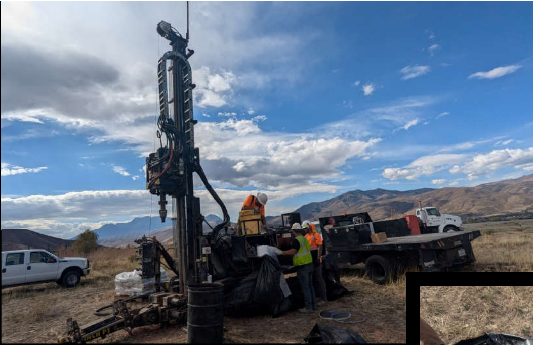
Drilling cores for soil testing. Start of the new runway project
