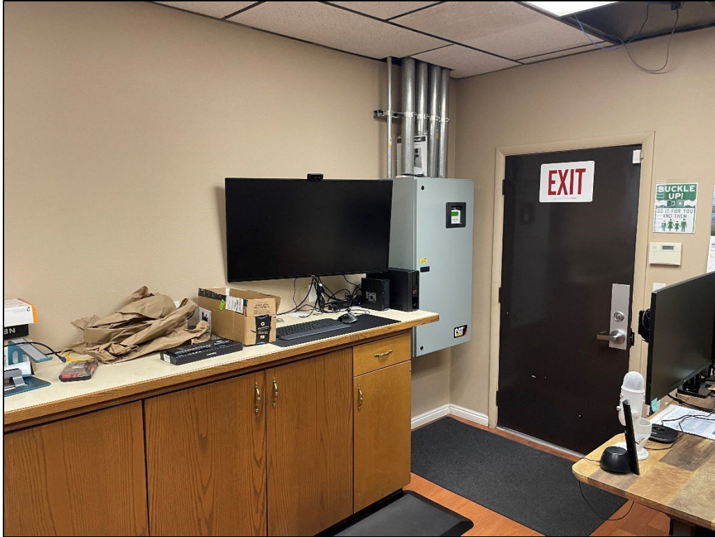
East Building Office Space
