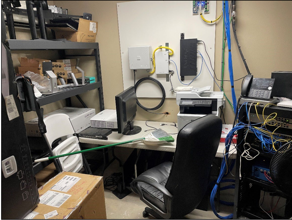
East Building Office Space
