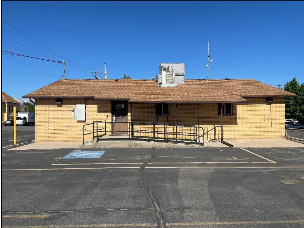
Main Building – East Elevation
