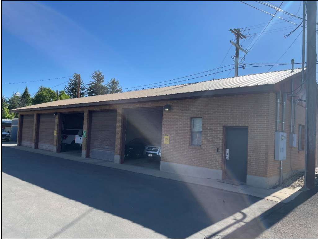
Front View of East Building
