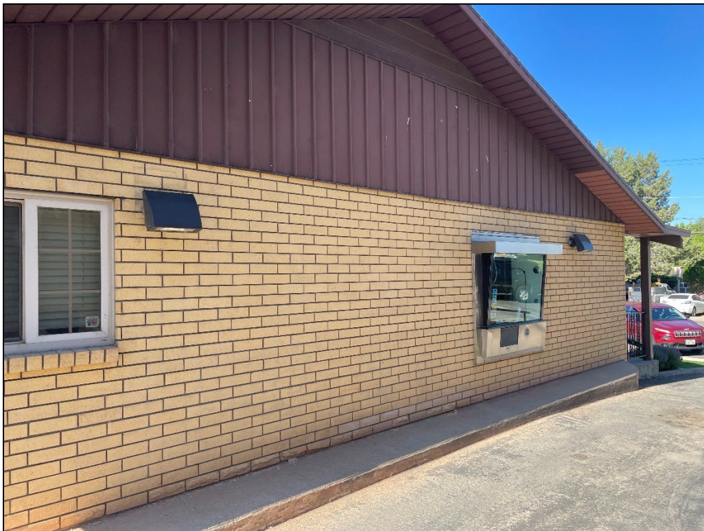
Main Building – North Elevation
